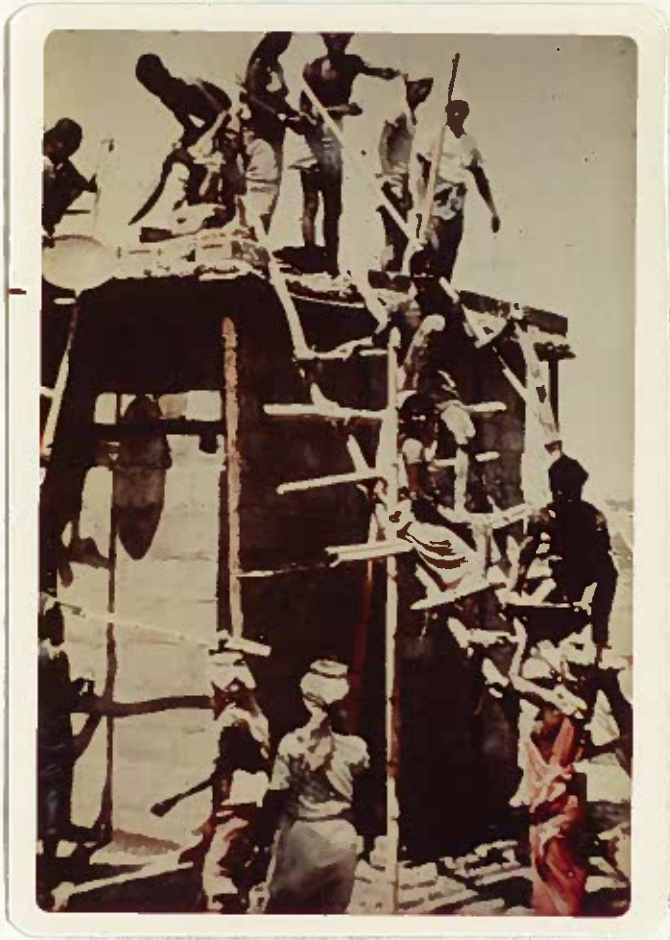
CONSTRUCTION IN INDIA
